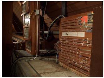
In addition to the above, all the so-called "primary valves" in the seven chests of the organ were releathered and completed refurbished. The old electro-mechanical relay switchboard was replaced by a new solid-state system and all electrical cabling was replaced. Two new rectifiers were installed in the organ chambers to convert incoming alternating current to the direct current needed to run the organ.
